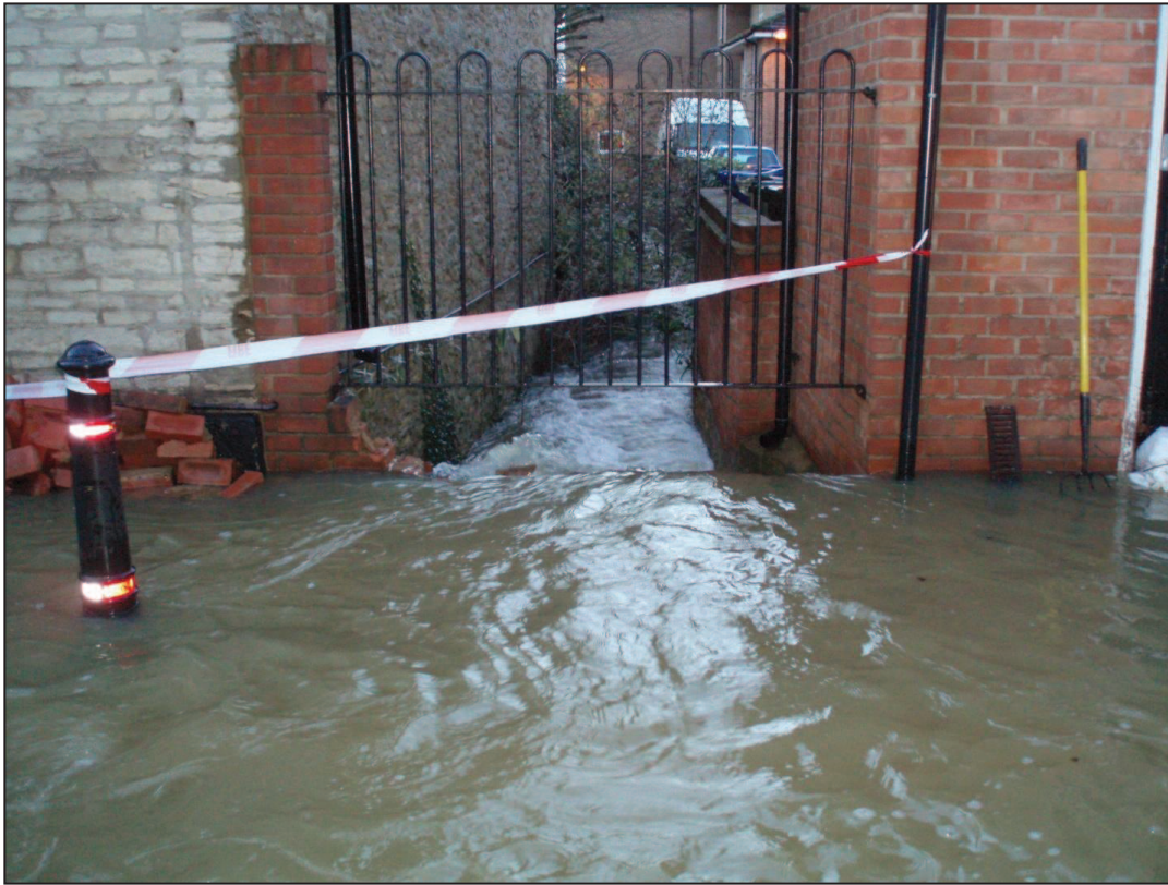
Figure 7: Section of wall removed on south side of Causeway by Oxfordshire Fire and Rescue Service to allow flood water to return to Back Brook
