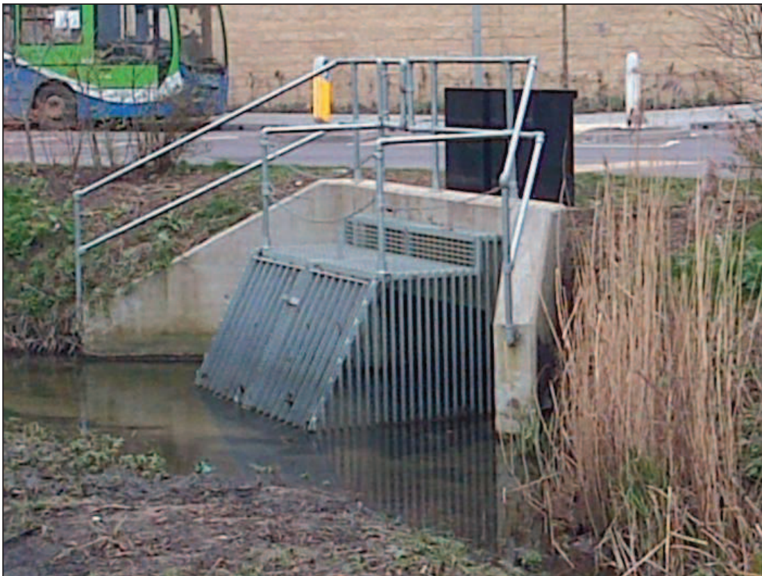
Figure 3: River Bure trash screen at Hanover Gardens during normal flows looking east
